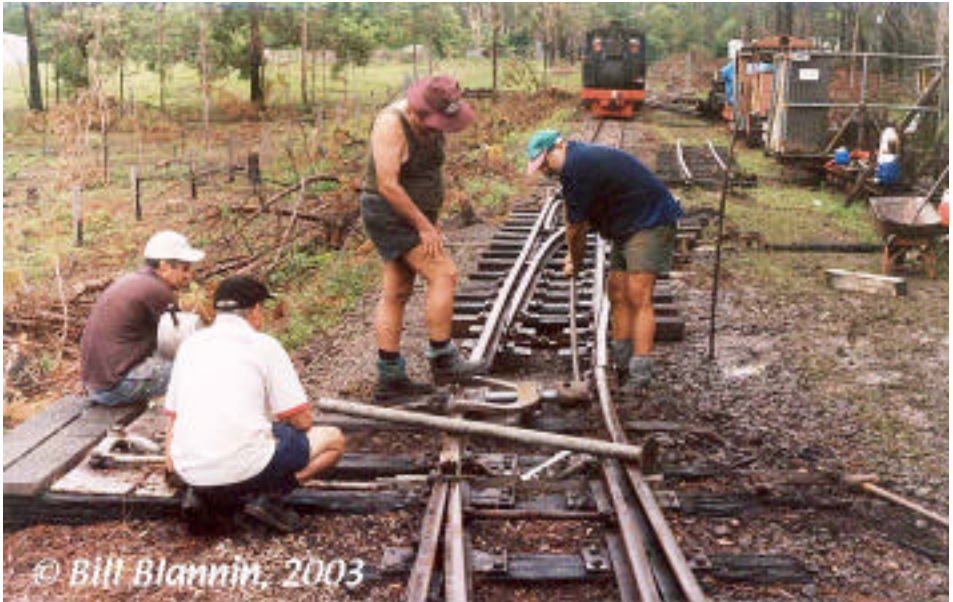
Saturday 22 nd February 2003. Greg Stephenson using the repaired rail bender to align the points with the existing track at the workshop end. Terry Olssen, Brian Wilson and Bob Gough assisting. Photo: Bill Blannin
