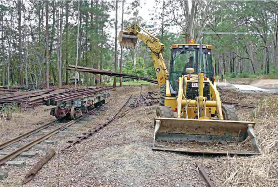
Ralph Cumner using his back-hoe to sort and load rails as part of the preparation works. To the right of the back-hoe, the new level crossing can be seen and, to the left, the wagon is on the existing mainline which needs to be connected to the level crossing. Below the rear bucket of the back-hoe are the points to become “S3” – these will be moved to connect immediately to the level crossing. Greg Stephenson photographer.
