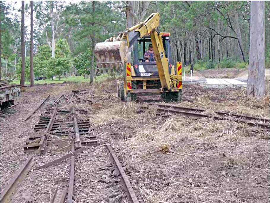
Moving welded panels of track out of the way. The back-hoe is standing where the future Storeybrook Station will be located. Greg Stephenson photographer.
