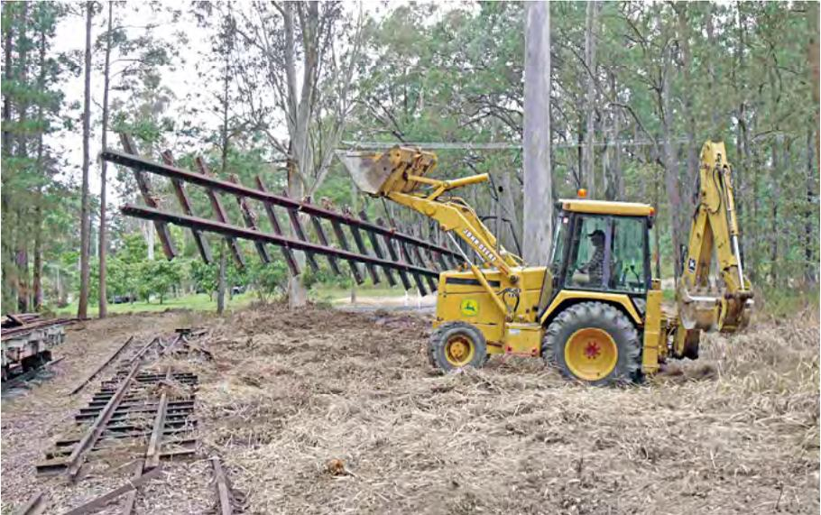
Ralph Cumner makes light work of moving a panel of welded track out of the way near Storeybrook Cottage. The tree behind the middle of the back-hoe marks the centre of the future mainline and needs to be removed. Greg Stephenson photographer.
