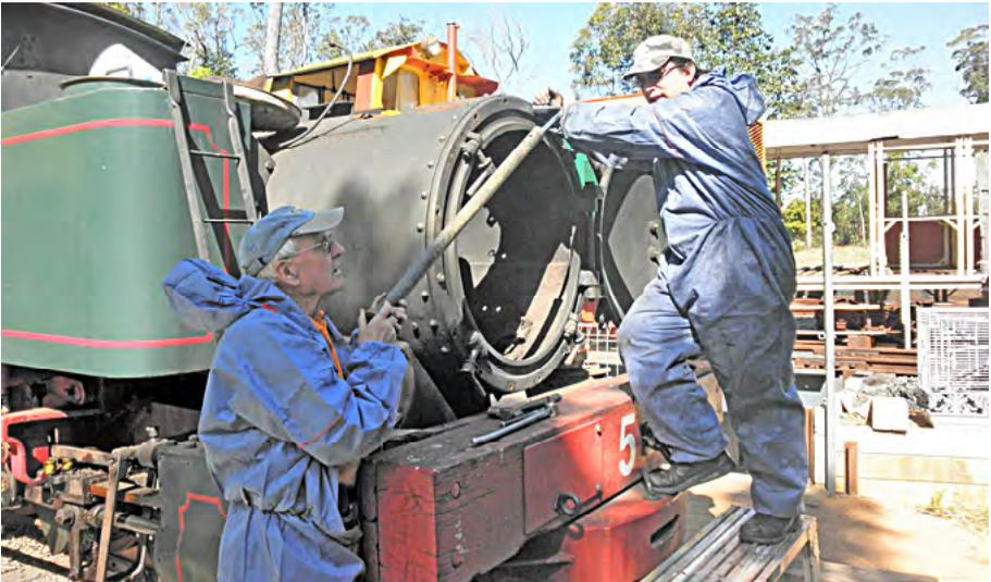
Bob Gough & Brad Bell removing rusty nuts & bolts from smoke box door ring on Bundy No 5. The ring & door were later removed to storage. Mark Gough photographer.
