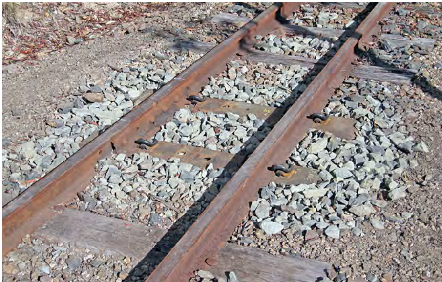
Special sleepers (above and below) for fishplate joints. Terry Olsson photographer.
