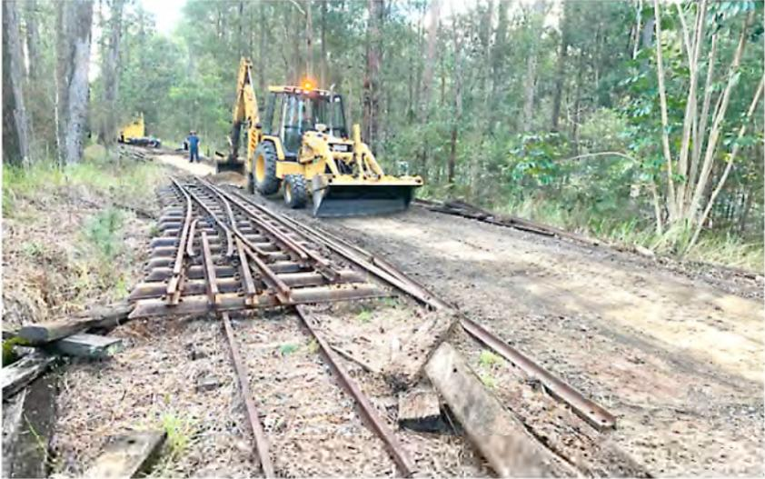
Above: With the existing ballast, sleepers and rails removed, Ralph Cumner is excavating the new ballast bed, 8 August 2020. To the right of the backhoe, the new points have been offloaded onto ground and await installation. Below: Looking towards Peterson Road, 15 August 2020. Two sets of points in place and reconnected to the existing mainline and awaiting ballasting. To the left can be seen the future passing loop for the new Peterson Road station. Ryan Thomas photographer.
