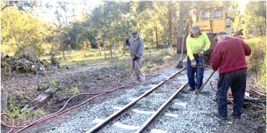
Packing, levelling and shaping ballast on an area of sleeper renewals at the start of Freeman's Cutting, Ryan Thomas photographer.
